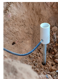
Ground-wire to Grounding Rod
